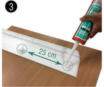
Apply DecoFix Hydro in V-Fix over the entire length
